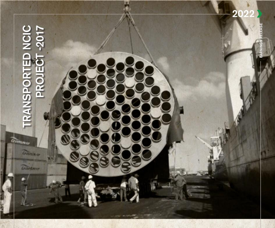
Egytrans discharged the highest drying tower in the NCIC project 9.75 m height 10.0 m width.
