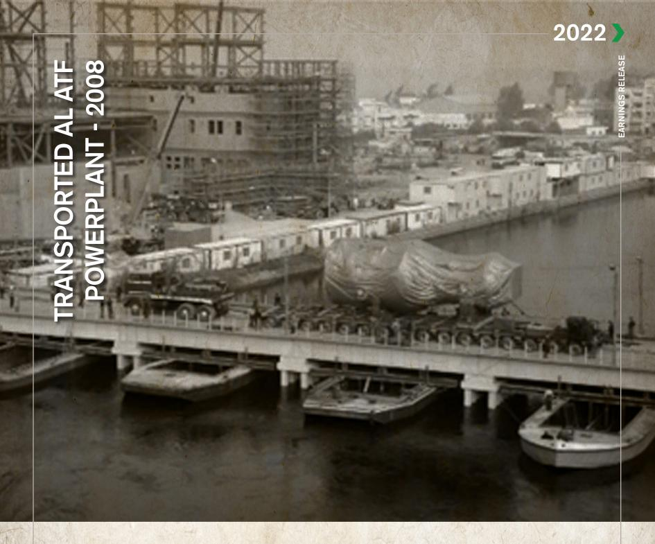
Transporting a gas turbine for Al Atf Power Plant after reinforcing Al Atf bridge due to the turbine's heavy weight of 372 tons.
